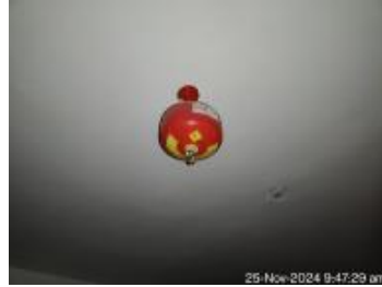
Mounted Ceiling Extinguisher.jpg
